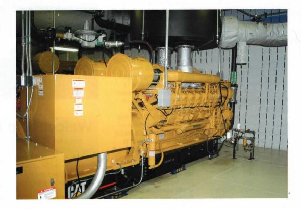
engines will be synchronized to deliver enough electricity to meet the needs of the entire campus in just two minutes. "We can bring an individual engine up in 20 seconds, but it can't carry the campus load, so we bring them all up and synchronize them before we throw the switch," says McCoy.
