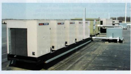
Only a small portion of the Roche campus is currently being cooled by the gas-fired absorbers. "Right now, I've got 5 of these machines, with 23 ammonia absorbers," McCoy says, adding that existing rooftop units will probably be replaced by gas-fired systems as they reach the end of their service lives.
